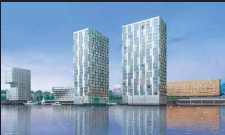
Almere. Side by Side (de Architecten Cie.)
